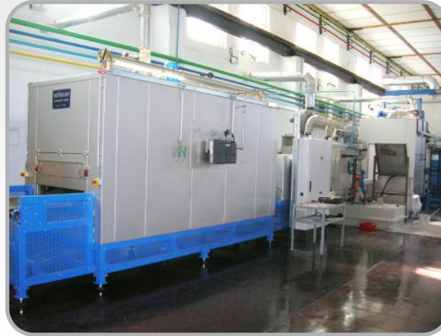
Installation of thermal degreasing - firm "Sellacan" (Germany)
